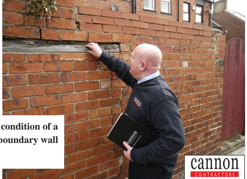
**Here is one of our surveyors inspecting the condition of a timber lintel in a boundary wall**
